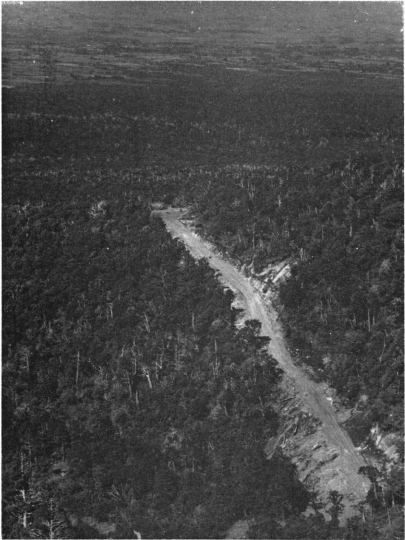
Egmont.—Road to the T.V. translator up the face of the Ngatoro Valley.
